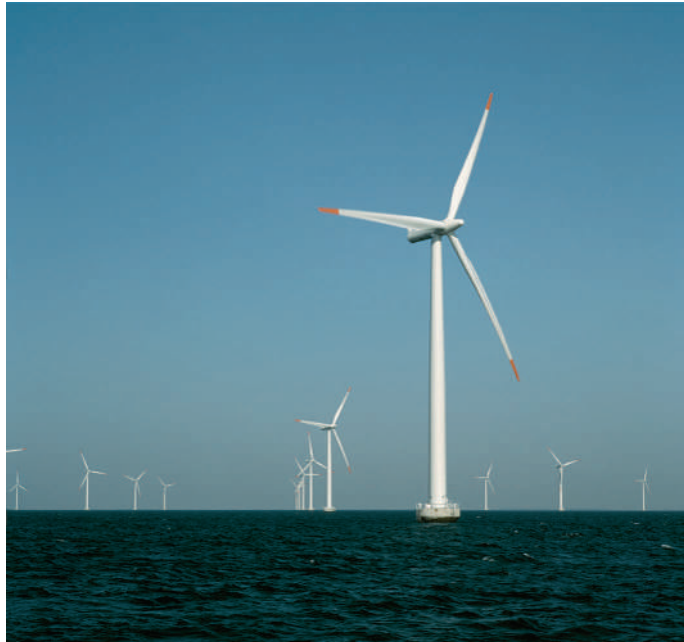
16 Application example, offshore wind turbine
